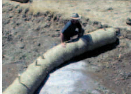
20" wattle in a swale
