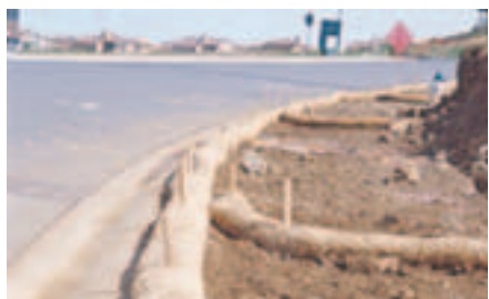
Prevent Construction Sedimentation
